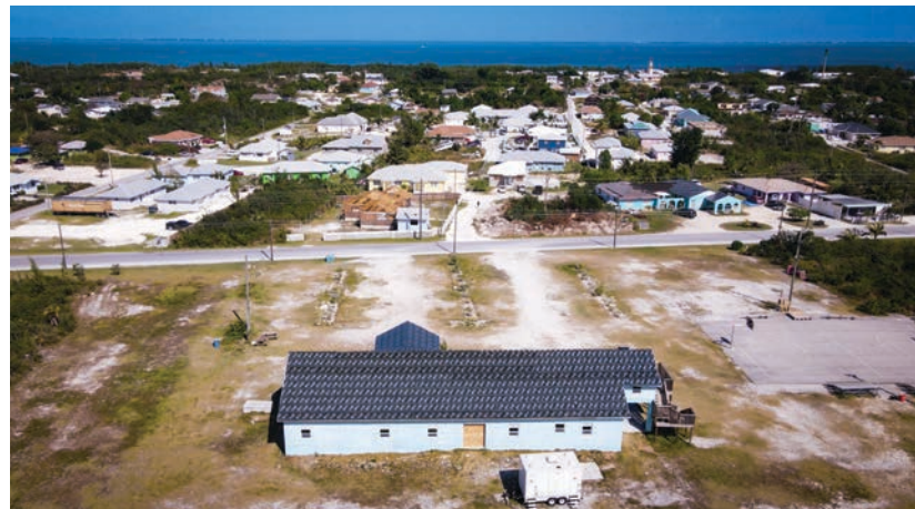
An aerial view of the Murphy Town Community Center under construction
